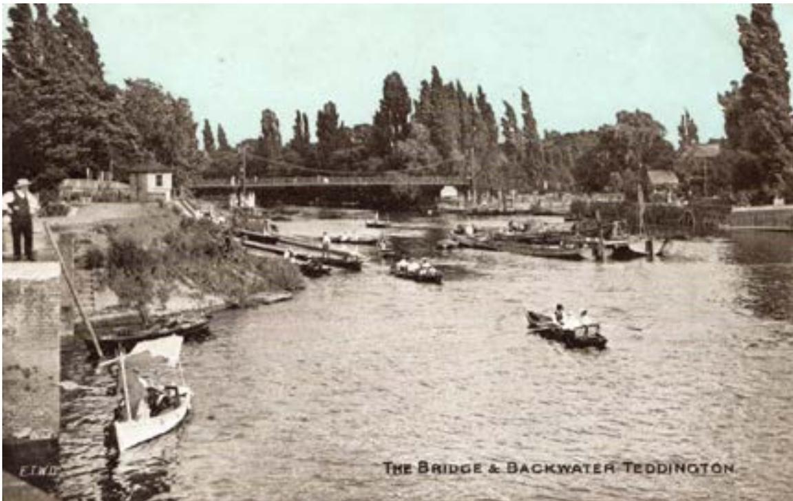
The two footbridges were built between 1887 and 1889, funded by donations from local residents and businesses. They replaced a ferry which gave its name to Ferry Road at Teddington. The northern bridge consists of a suspension bridge crossing the weir stream and linking the island to Teddington. The southern bridge is an iron girder bridge crossing the lock cut and linking the island to Ham on the Surrey bank.
